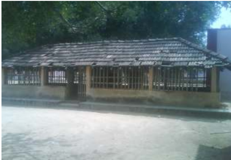
Partially Pucca School Building
