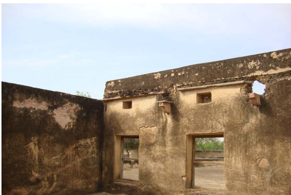
Condition of School Building
