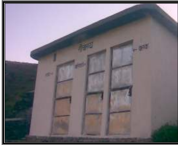
Picture - Toilet in Pipalkot
